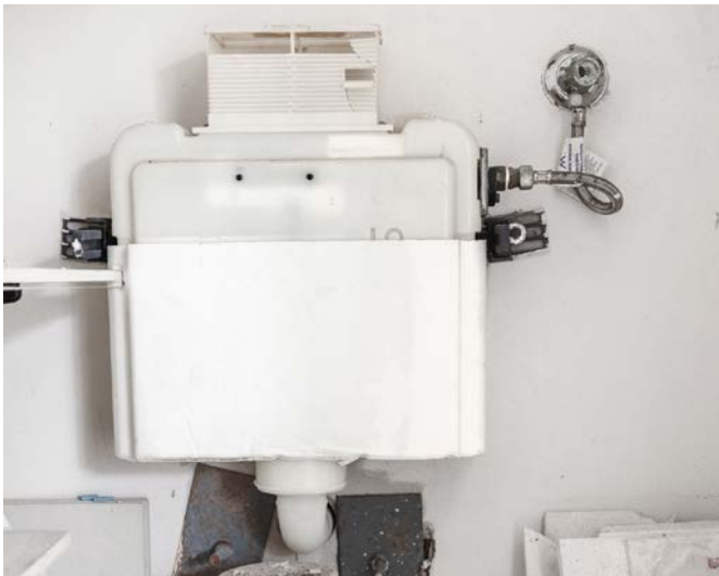
Geberit concealed cistern installation
