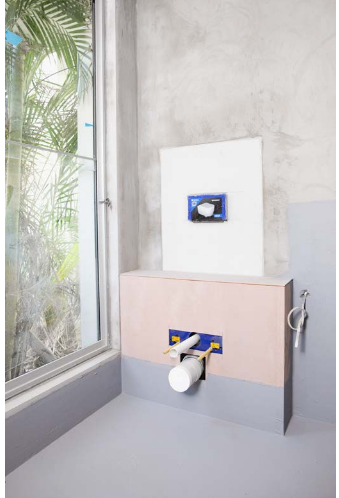
Geberit concealed cistern installation
